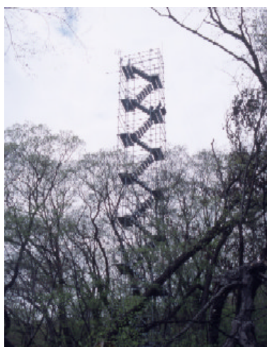
Fig. 2 Original flux tower built in 1999. Nowadays the part above canopy layer was removed and the flux measurement system moved to the main tower in late 2002. The tower is mainly used for various ecophysiological studies.
