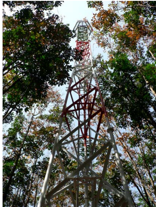
Fig. 4. The 25 m high, self standing tower, view at leaf-shedding.
