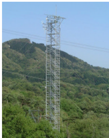
Observation tower located on the ridge
