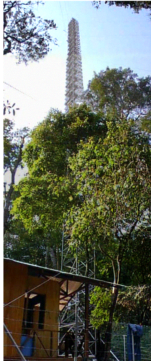
Fig.2 50-m meteorological observation tower in Kog-Ma watershed, northern Thailand
