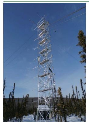
**Fig. 3.** The 17m scaffold tower for eddy covariance and micrometeorological measurements in the black spruce forest in the property of the Poker Flat Research Range.
